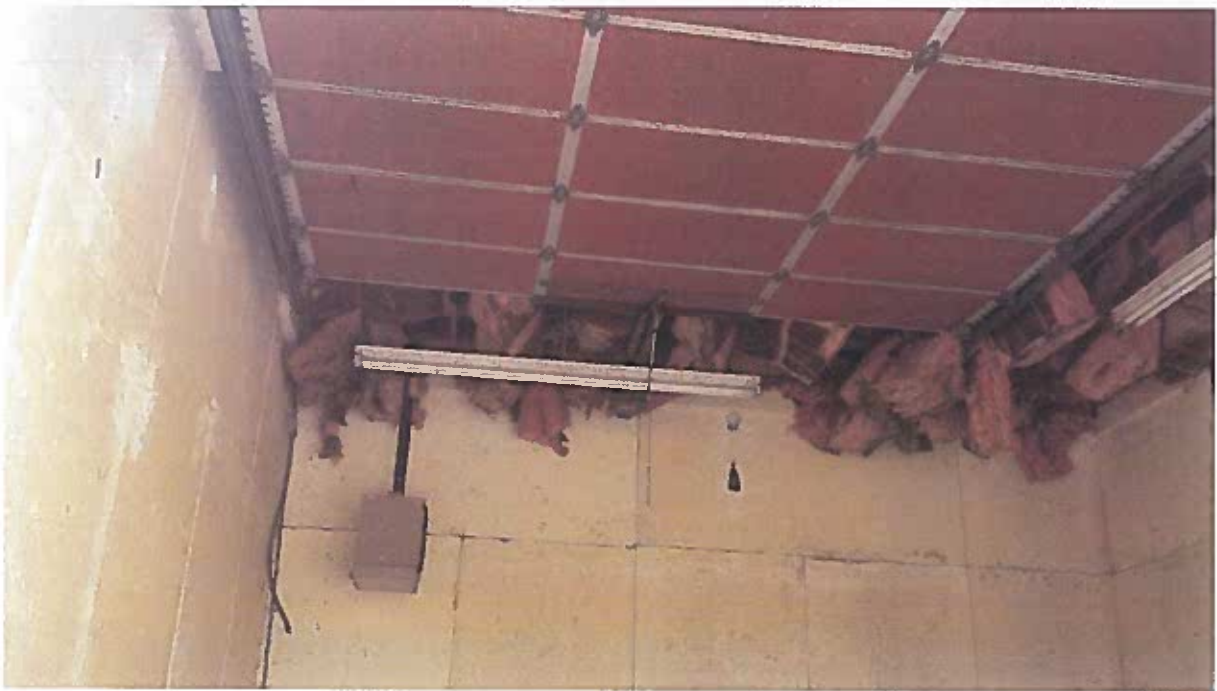
Ceiling Damage- Significant Roof Failure
