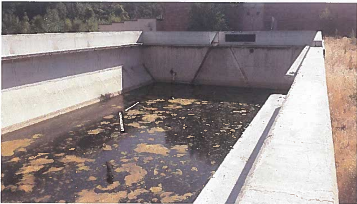
Concrete Sediment Holding Tank
