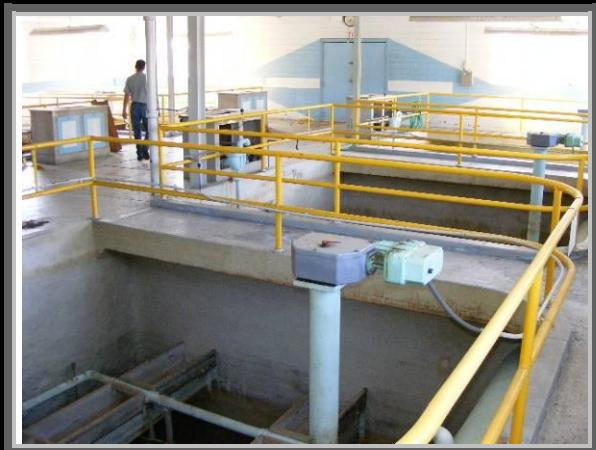
Photograph 19: Filter Room - contains six filter chambers, located in the central portion of the South Plant.
