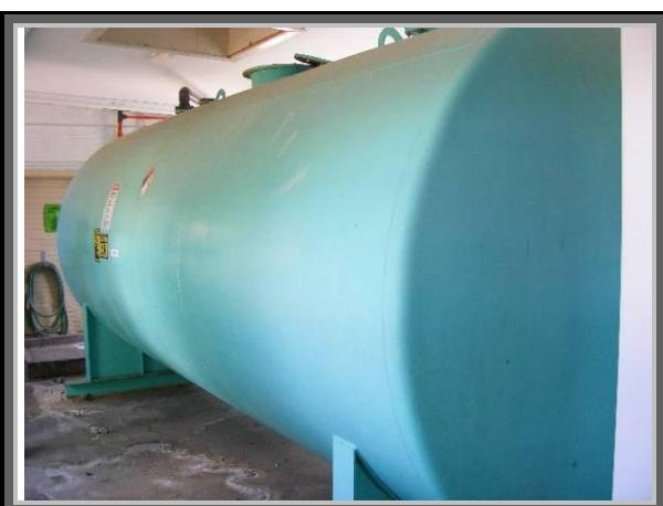
Photograph 17: 6,000 gal metal AST for Aluminum Sulfate located in the Chemical Mixing Bld. in the western portion of the South Plant.
