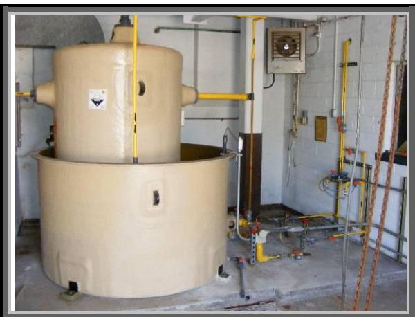
Photograph 15: Bleach/Chlorine storage room located in the basement of the Main Building.
