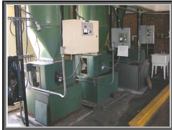
Photograph 22: Hoppers for inducing Soda Ash, Sodium Fluoride, and Activated Carbon, located in the upper level of the Main Bld.
