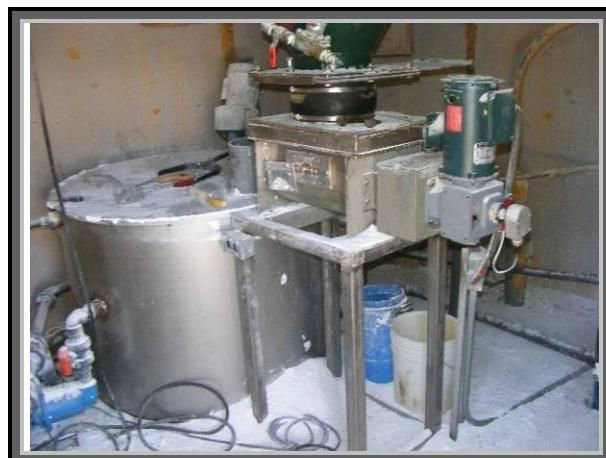
Photograph 28: View of vacuum system inside the Soda Ash Silo located in the eastern portion of the site.
