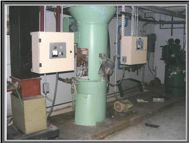
Photograph 17: View of dry chemical hoppers in lower level of Chemical Mixing Room.
