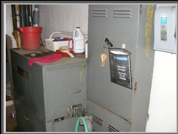
Photograph 23: View of the elevator controls and hydraulic fluid reservoir located in the basement of the South Plant Main Building.
