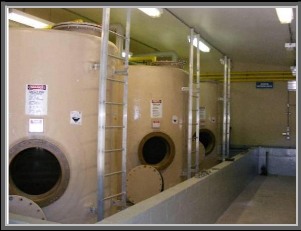
Photograph 22: Approx. 4,000 gal metal ASTs for Bleach located in the Bleach/Chlorine Bld. in the central portion of the North Plant.
