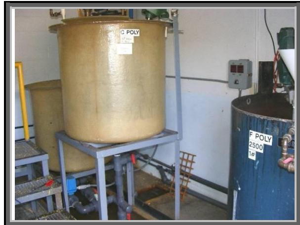
Photograph 18: Mixing tanks for coagulation and flocculation polymers, located in lower level of Chemical Mixing Room.
