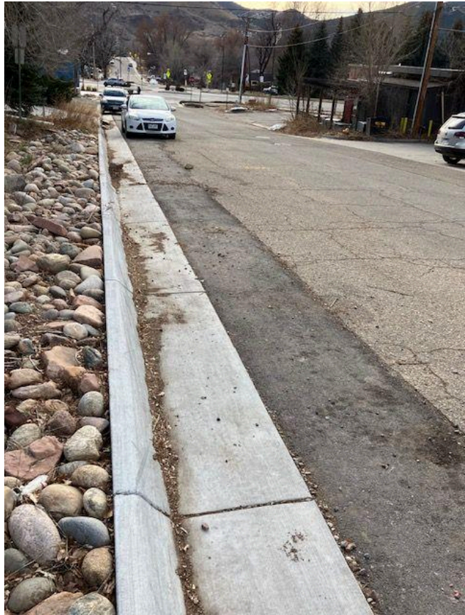
Photo 11 – Temporary (?) curb & gutter on west edge just above Kelling Dr. to address prior deep erosion.
