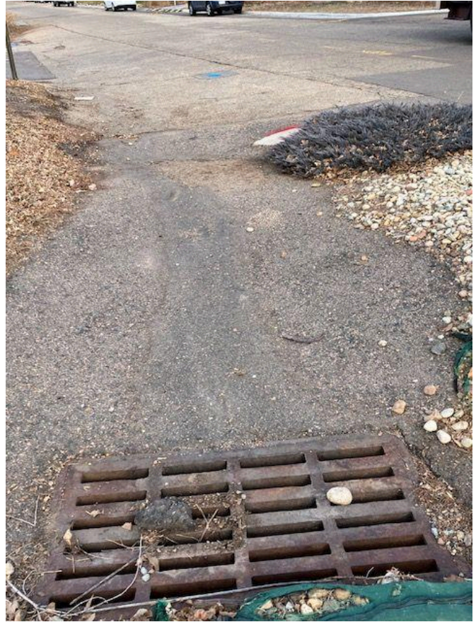
Photo 7 – Stormwater catchment basin at lower west end is < 3 feet deep. (Note washed-down asphalt piece on cover.)
