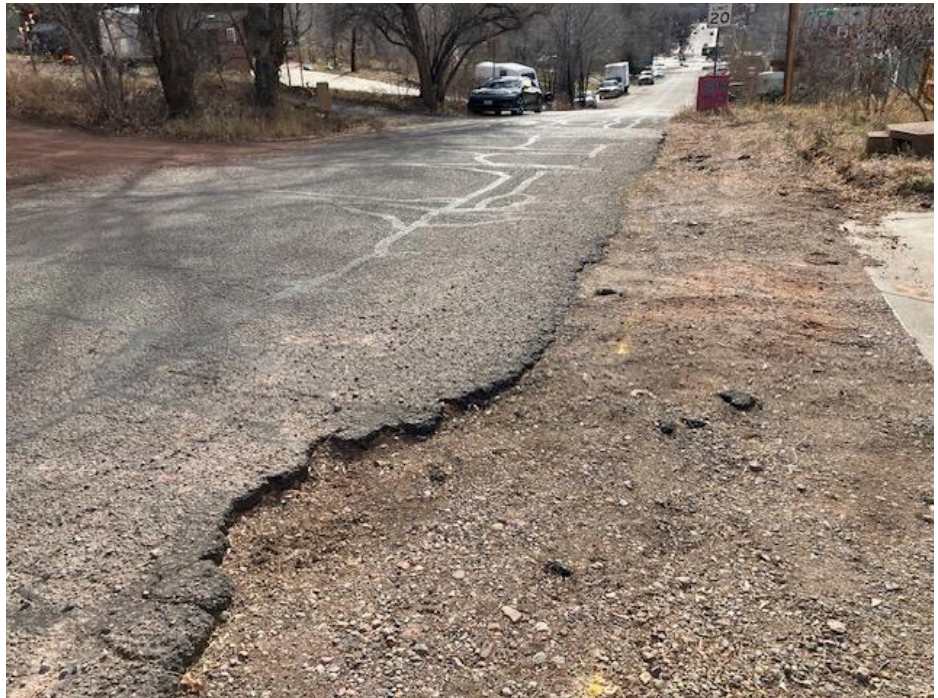
Photo 3 – Another area (between High & Old Main) narrowed to 21 feet by washed-out asphalt
