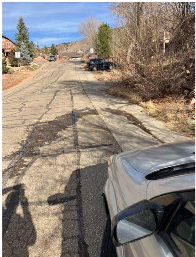
Photo 8 – 6' concrete swale on east side extends from between Old Main & High to above 1st Ave. Concrete is in decent shape.
